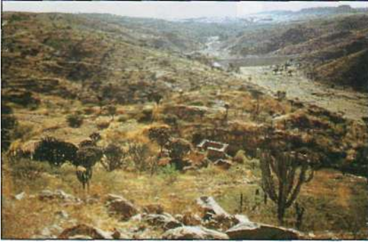
Euphorbia and a dam under construction
