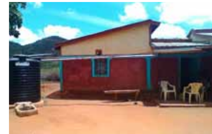
Photo 2: Roof water harvesting in Kwa Vonza, Kitui County (Photo credit: MetaMeta)
