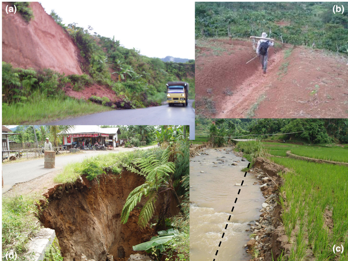
Fig. 8. Landsliding next to the main road north of Bukit Rigis; b) Footpath erosion in the Way Ringkih (WR) catchment on the northern slope of Bukit Rigis; c) River bank erosion of the Way Petai (WP) after the storm of 14 January 2005. The dotted line illustrates where the river bank was before the storm; d) Gully erosion in Sumberjaya.
