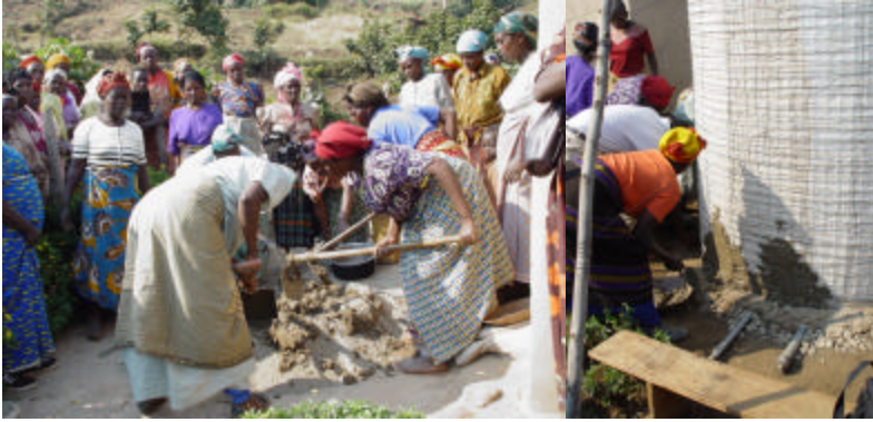
Plate 3 Women constructing a Ferro-cement tank in Kabale, Uganda
