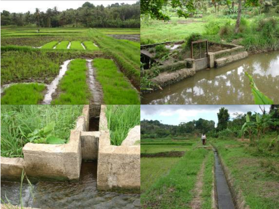
Plate 6 River diversion and surface irrigation in Pemba (Photos by Maimbo M. Malesu 2007)
