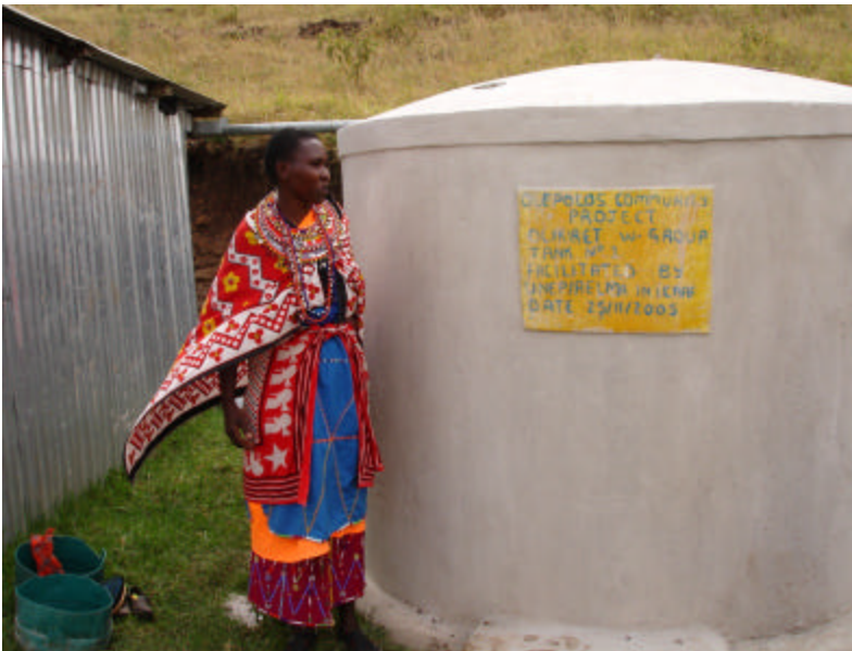
Plate 4 Proud owner of Ferro-cement tank in Kajiado, Kenya
