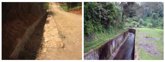
Figure 12-3: Concrete lined cut-off drains in Kapingazi, Embu Kenya.<sup>35</sup>
