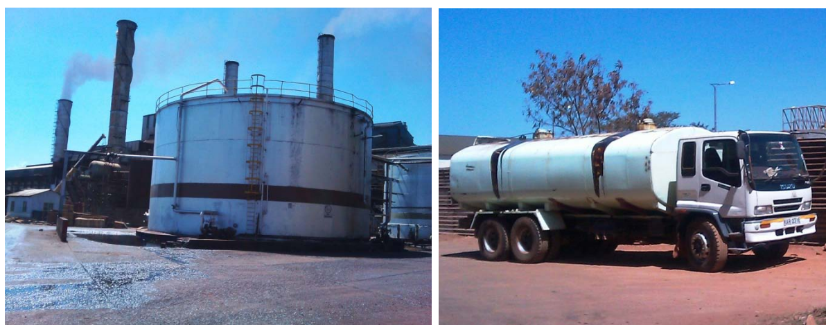
Fig. 15: Molasses storage tank (Right) and Molasses transportation tank in Mumias sugar
